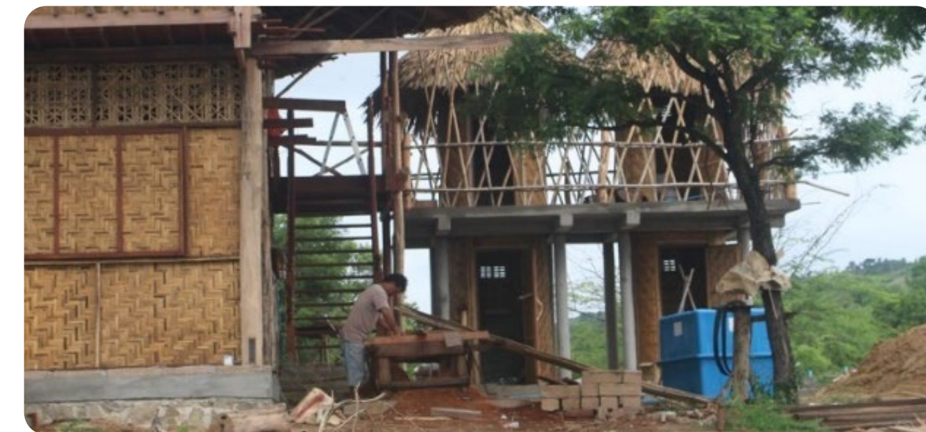
Newly constructed training hall in Myaing CBT
