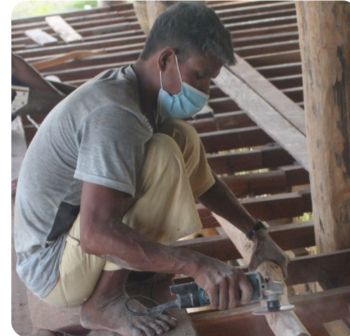
Ko Than Htike working in a construction site
